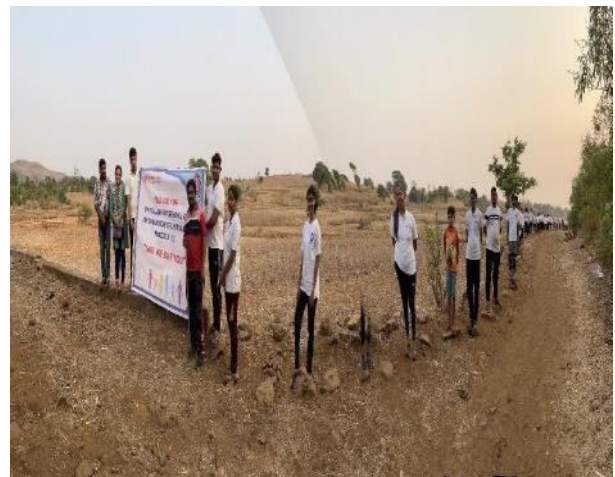
NAME OF THE ACTIVITY: Repairing of Raw Road (Sadak)& Creating a pathway to Farm at Adopted Village Palsunde DATE: 20th March 2022 to 26th March 2022 TIME: 10.00 AM TO 5.00 PM Venue: Palsunde, Mokhada
